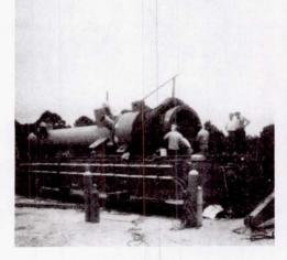
Figure 5A Top Bearing Housing & Pivot Column Being Assembled
