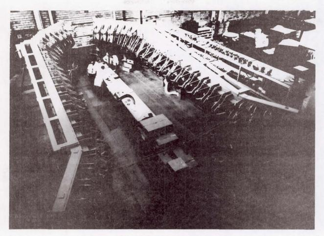
FIGURE 10.- WING LEADING EDGE FINAL ASSEMBLY FIXTURE.
