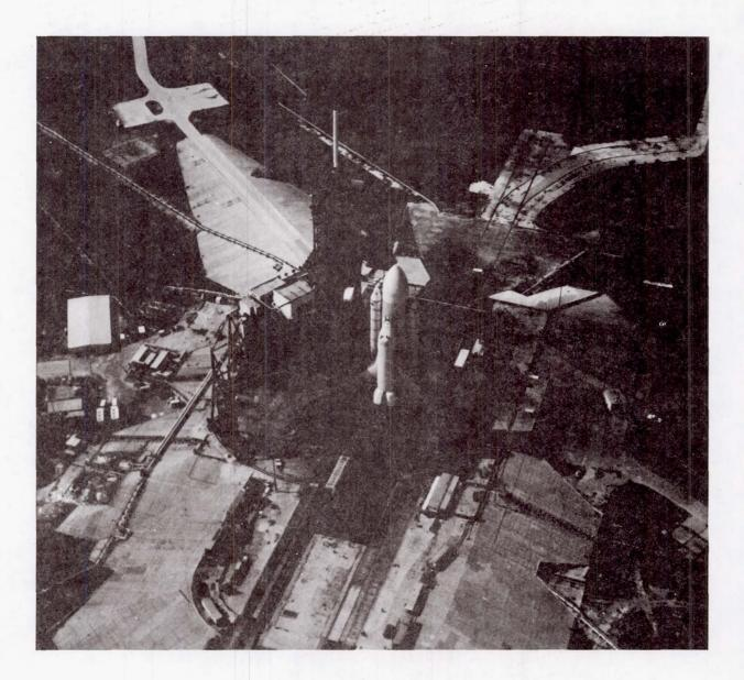
FIGURE 1. ROTATING SERVICE STRUCTURE SHOWN IN RETRACTED POSITION - SHUTTLE READY FOR LAUNCH
